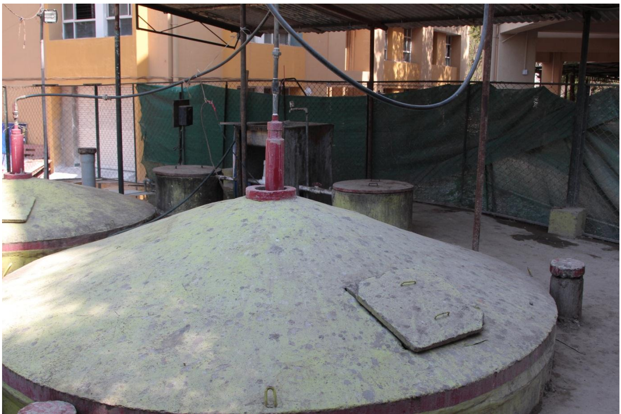
Bio Gas Management System
